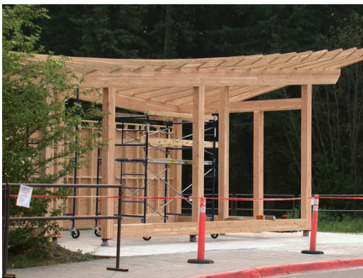
Figure 2.9 UNBC Bus Shelter Under Construction
