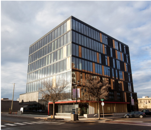
Figure 2.18 Wood Innovation and Design Centre
